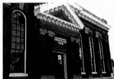
Renovated Galveston Water & Electric Light Building
